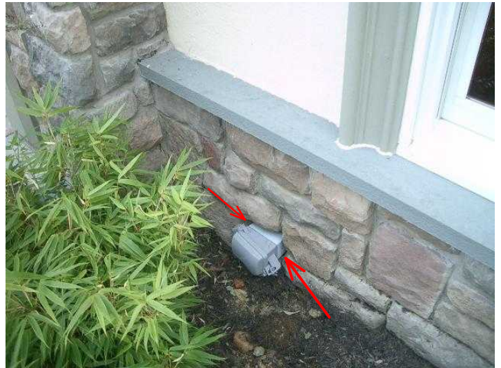
Exterior Outlet---seal around box
