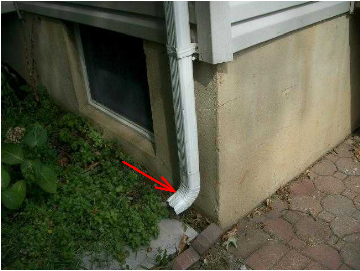
Downspouts-----extend away from foundation
