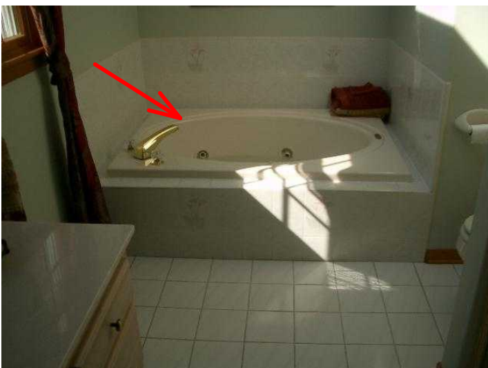
Master Bath---2 floor, tub working at time of inspection
